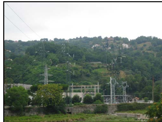
Area 26 –centrale ENEL -
