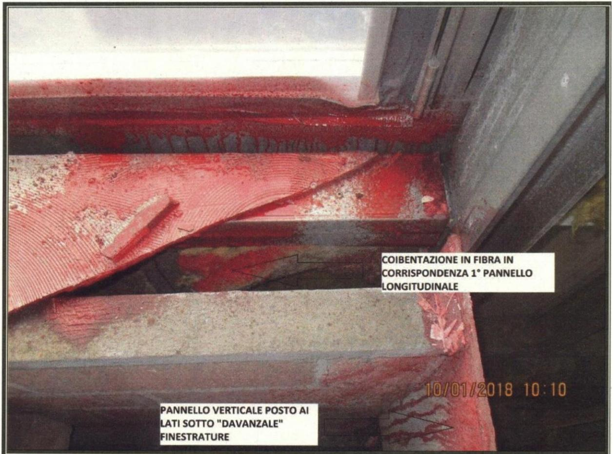
FOTO N.14: LANA MINERALE PERICOLOSA E PANNELLI PERPENDICOLARI ALLA FACCIATA
