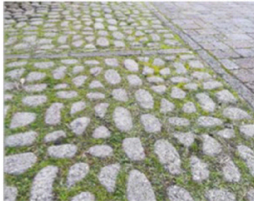
1. Draining pavement (photo: K. Perini)
