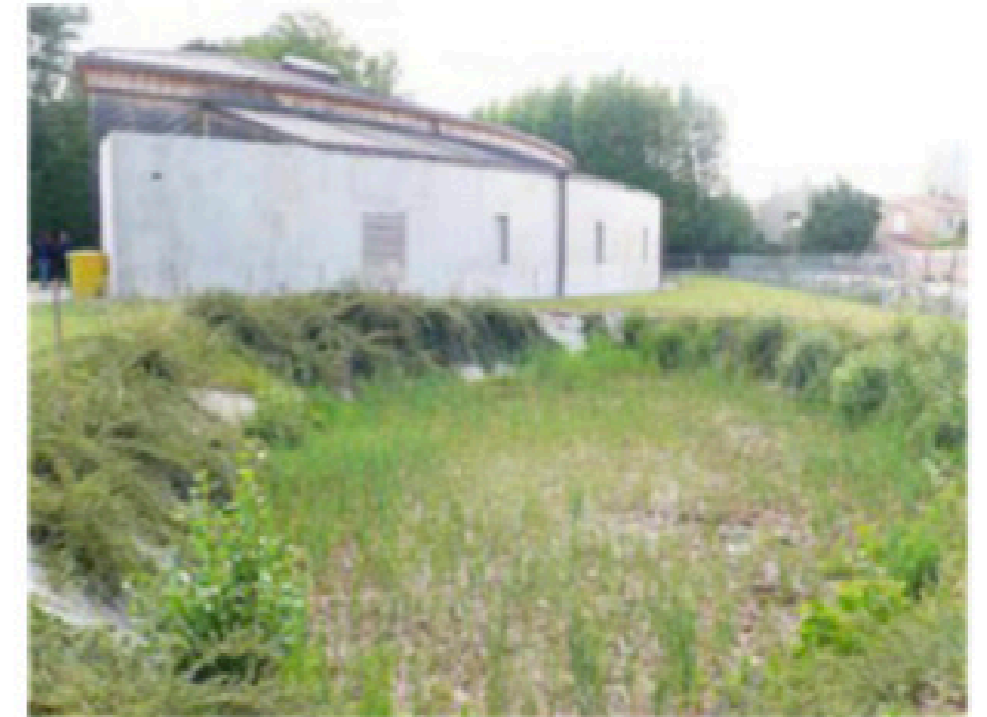
2. Infiltration basin (photo: K. Perini)
